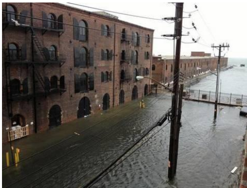
FLOODING IN RED HOOK AFTER HURRICANE SANDY
